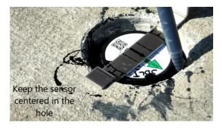
When the sealant is cured, detach the tool from the Pod by pulling up on the tool. The tape will peel away from the Pod housing.
